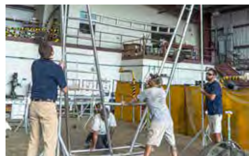
Brett, Sam "Wally" Smith, Mike Houghton and Curtis Updike (left to right) raise the tower aft section ladder so the front leg can be welded to the ring.
