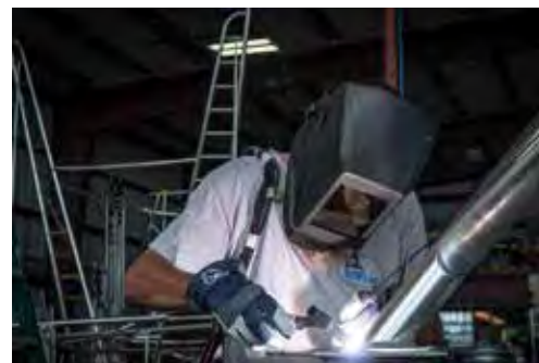
Welder and Fabricator John Lindgren welds out the front tower leg section, between the tower ring and platform, before installing it back to the tower.
